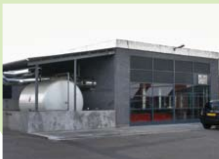
Heating central with gasoil tank ash container.
